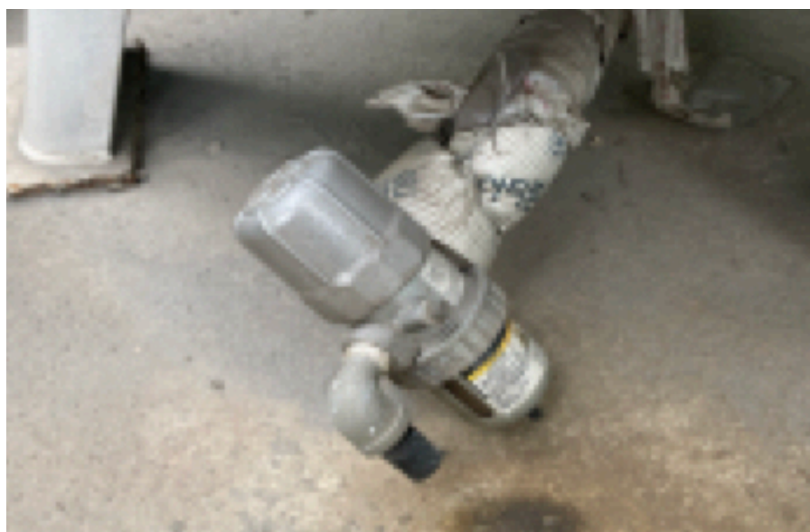
Receiver Tank Drain Trap
