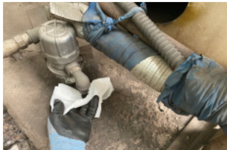
Receiver Tank Drain Trap
