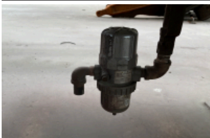
Tank Drain Trap
