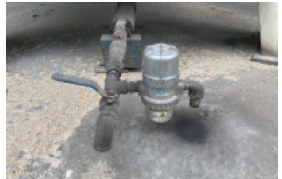
Receiver Tank Drain Trap
